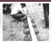
3a. The concrete bedding method\* requires a stiff concrete bedding slurry (somewhat dry) along the length of the trench. The bedding concrete should be as thick as the floor or driveway. Butt the channels together in the trench, on top of the concrete. Allow the concrete bedding to cover approximately 2" up the side of the channel. Align the top of the channel with the string line. Allow the concrete bedding to set. Connect the outlet piping as required.
