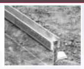
1. Dig a trench 12" to 18" wide and at least 8" deep. Set a string line to grade (finished elevation) the length of the PolySelf drain line.
